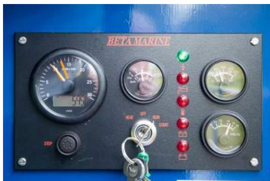
Press the STOP button on the instrument panel.
