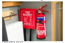
The fire blanket and extinguisher are located close to the cooker for use in an emergency. A further extinguisher is located close to each front and back door.
